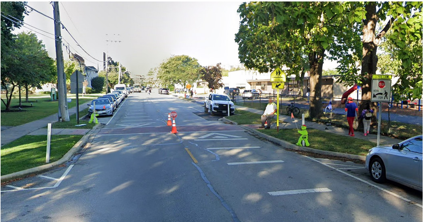
Existing crossing enhancements and traffic calming measures along Thacker Street near Central Elementary School
