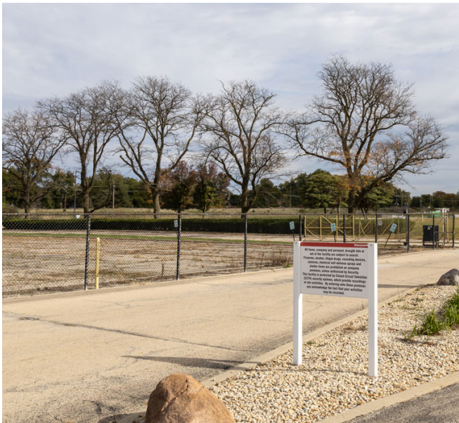
The future Seefried Industrial logistics site at 1055 S Mt. Prospect Rd.
