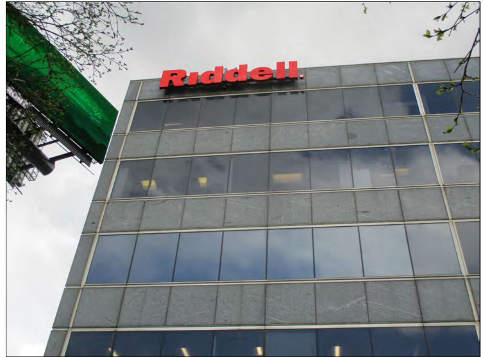
1700 W. Higgins Road – Existing North Tollway Wall Sign
